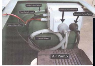
The warning light activates; If there is low air pressure (the air pump has failed, there is a broken pipe- or the sludge or skimmer control taps are wide open)
